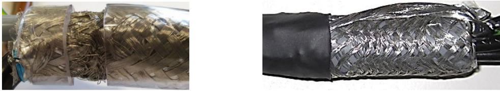
2. Determine the needed length of the wires, strip the cable and mount the cable lugs. Note that due to the touch protection of the cover, the wires need to be a little longer.
