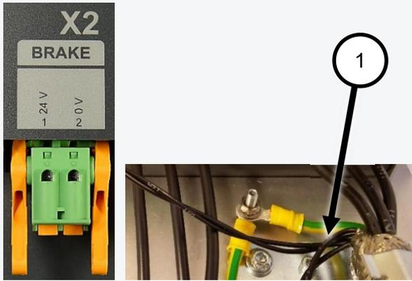
Connect the brake wires to the IMD X2 BRAKE connectors according to the wiring diagram and the instructions in section [5.2.2](#) on page [28](#).
