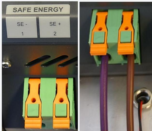
Connect the battery or Ultra Cap wires to the IMD X1 SAFE ENERGY connectors according to the wiring diagram and the instructions in section [5.2.1](#) on page [28](#).
