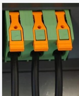
Connect the Mains wires to the IMD X1 MAINS connectors according to the wiring diagram and the instructions in section [5.2.1](#) on page [28](#).
